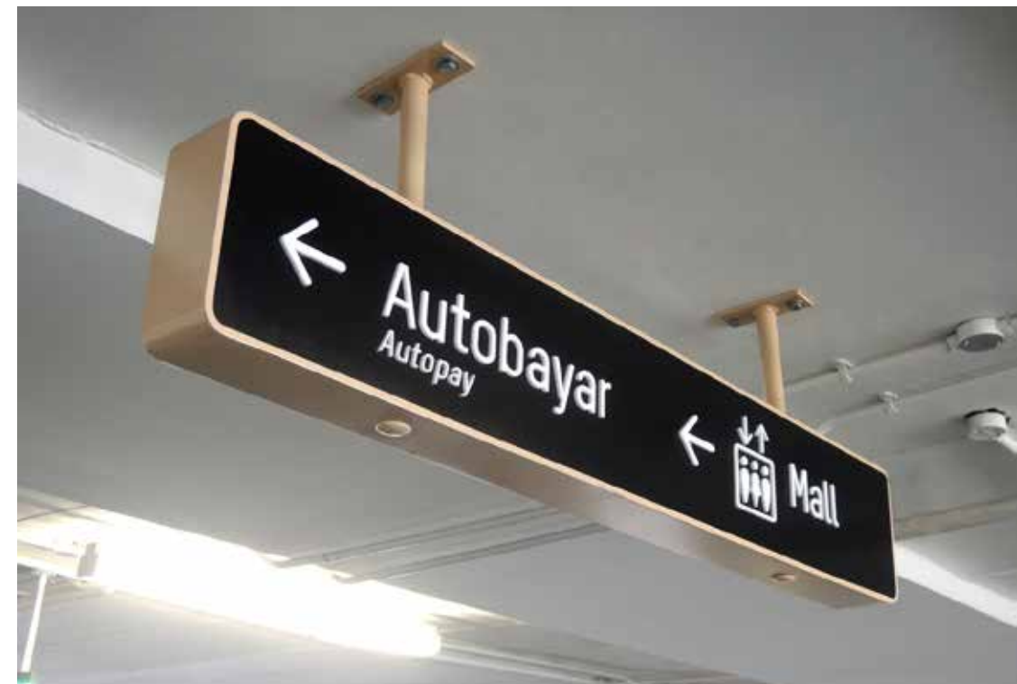
Our work continues after installation, with a defects report, rectifying the sign fabricator's work that did not follow specifications (e.g. the unsightly bolts in the photo above) and any additional signs based on visitors' and tenants' feedback.
